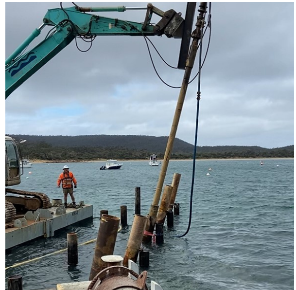
Coles Bay Jetty Extension - Pile Drilling
