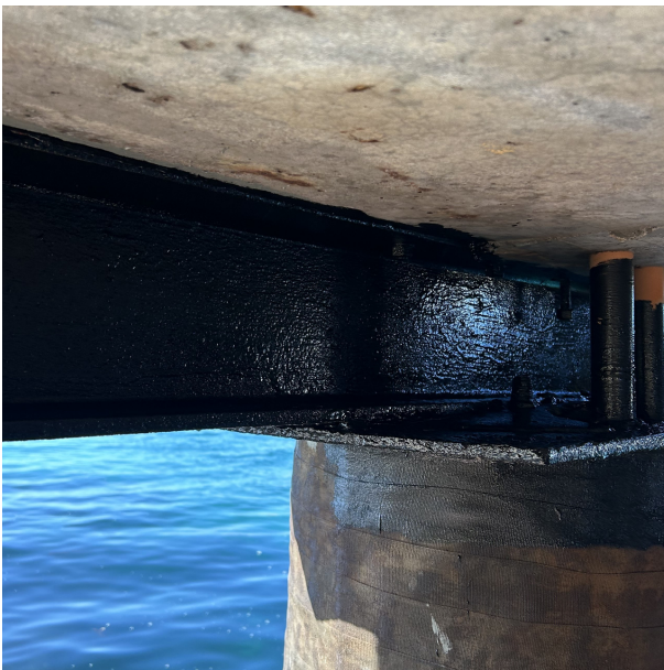
Bicheno Landing Stage - Coating
