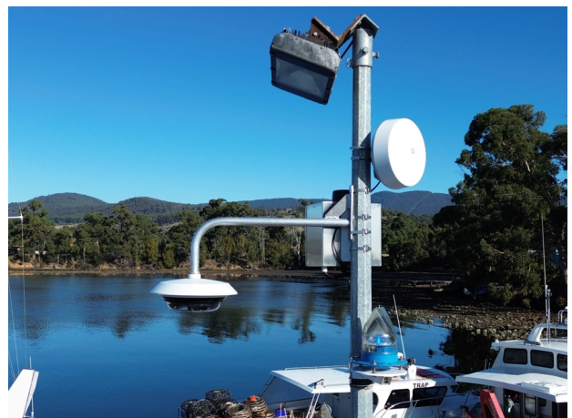
New camera installed at Margate Jetty
