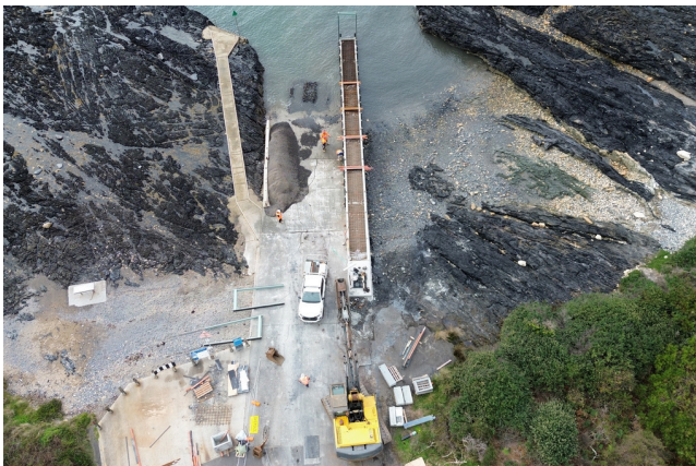
Works are underway at Sisters Beach boat ramp
